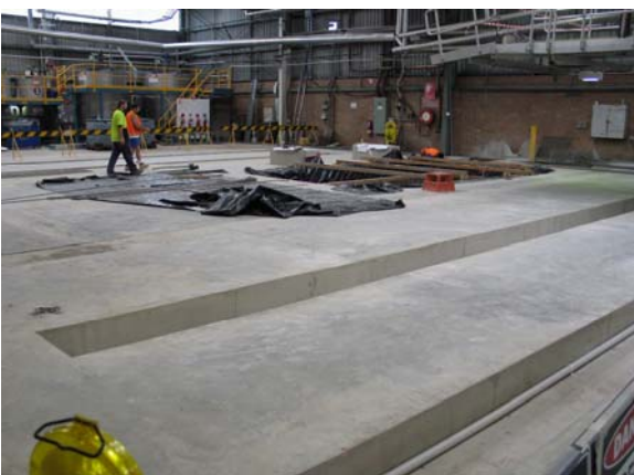
The concrete slab completed
