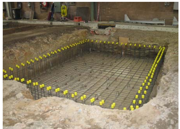
The steel reinforcement to the slab supporting the concrete plinth
