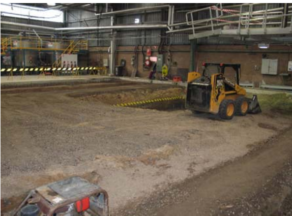
Ready for the concreting
