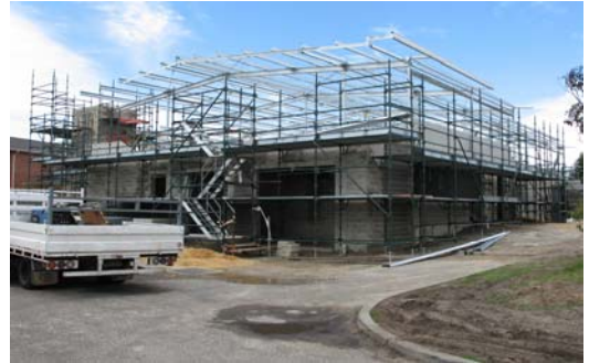
December 2004 - The steelwork underway.
