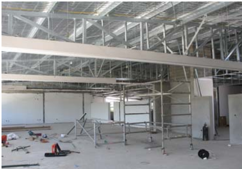
February 2005 - The fitout for upper level classrooms.
