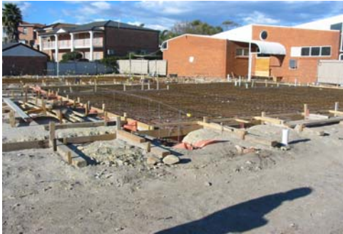
August 2004 - The foundation slab prior to pouring.
