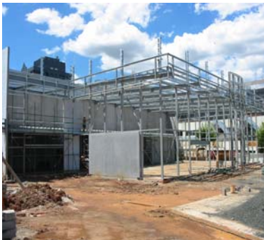
Structural steel inspection Late November 2004 - structural steelwork is nearing completion
