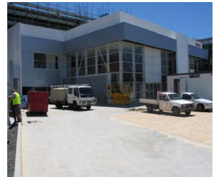
Final inspection Early February 2005 - The building nearing completion
