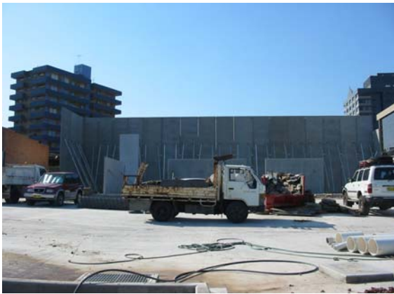
Early November 2004 - the panels had been lifted into position
