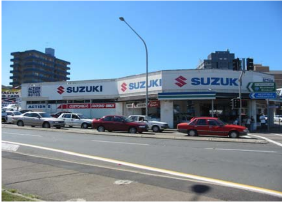
February 2004 - prior to demolition
