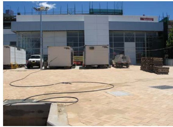
Early February 2005 – nearing completion
