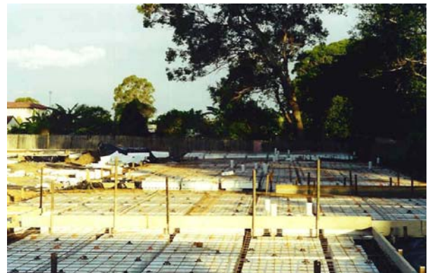
The waffle pods and steel prior to pouring
