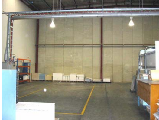
a) Before – Main wall before opening cut.
