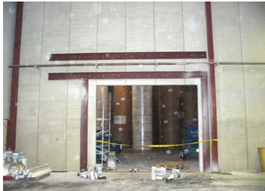
c) After - Main wall after opening cut.
