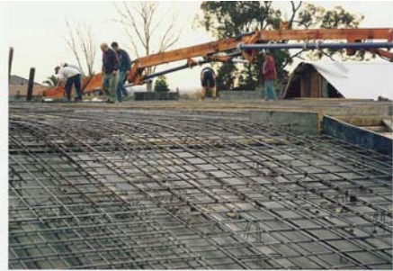
The steel reinforcement to the suspended concrete slab prior to pouring
