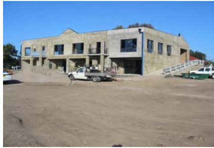
The building during construction
