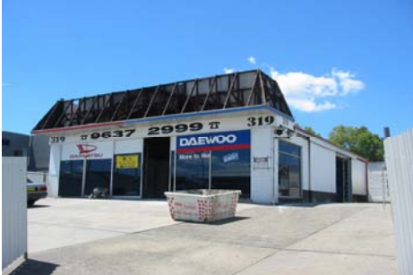
Outside at beginning of refurbishment
