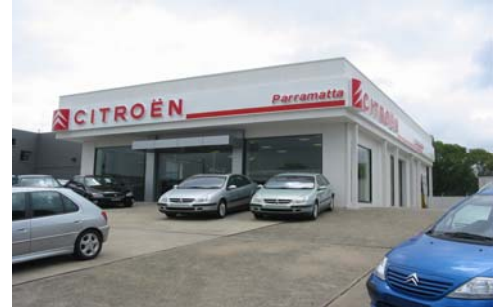
The outside after refurbishment
