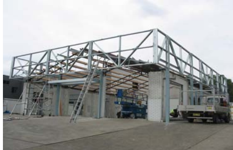
The structural steel during refurbishment
