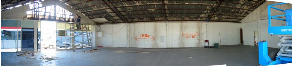
Inside at beginning of refurbishment
