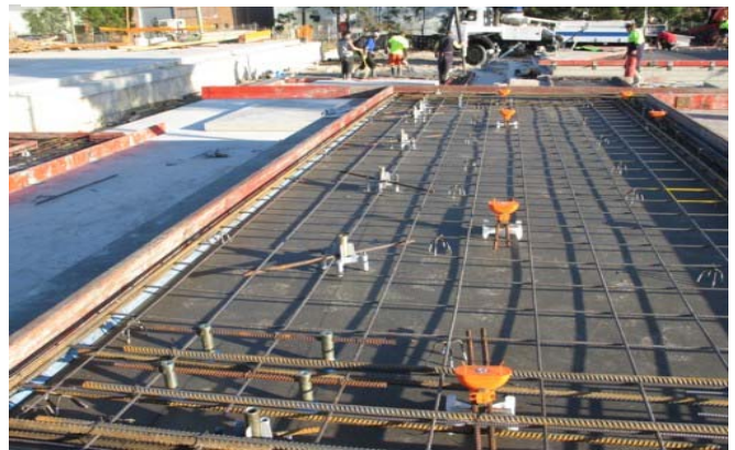
One of the many tilt up panels just before pouring.
