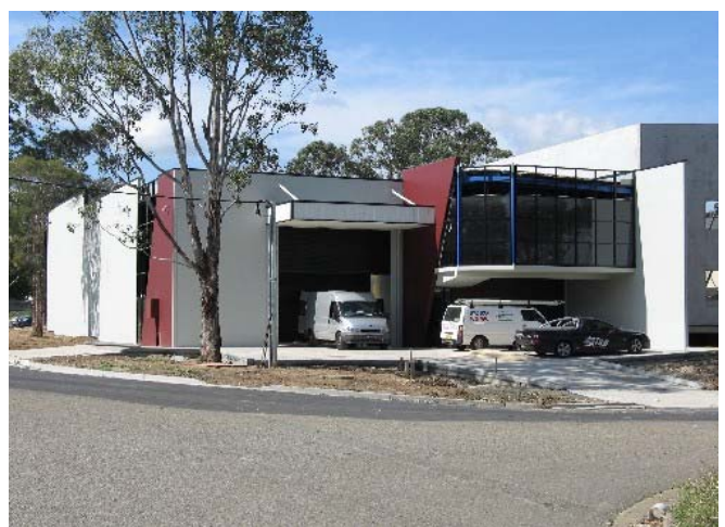
One of the two identical units nearing completion.
