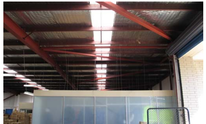
Some of the steelwork installed behind the façade
