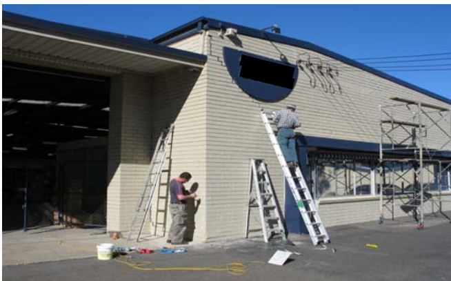
The front façade cosmetic repairs in action
