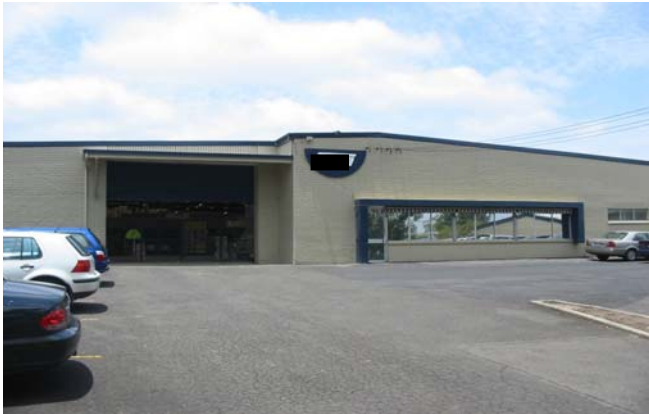
The front façade before repairs
