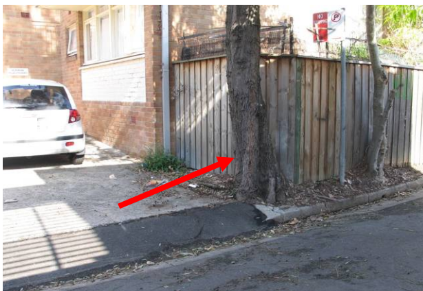
Proximity of tree to the fence and building
