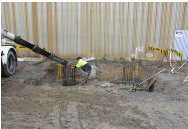
Pouring of the piers to the footing
