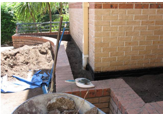
Nearing completion – ready to add plants.
