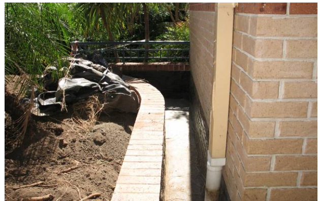
The planter box ready for re-waterproofing.
